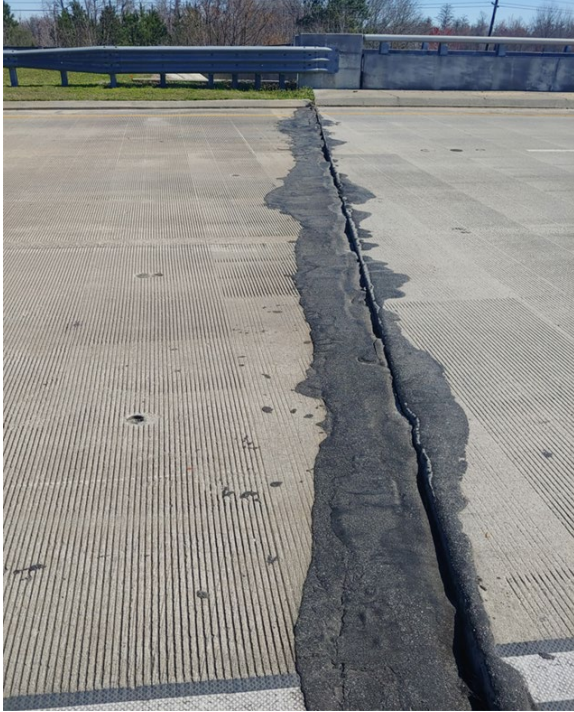
Approach Slab Repair
