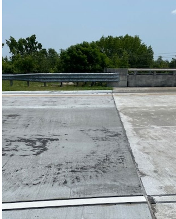
Approach Slab Repair
