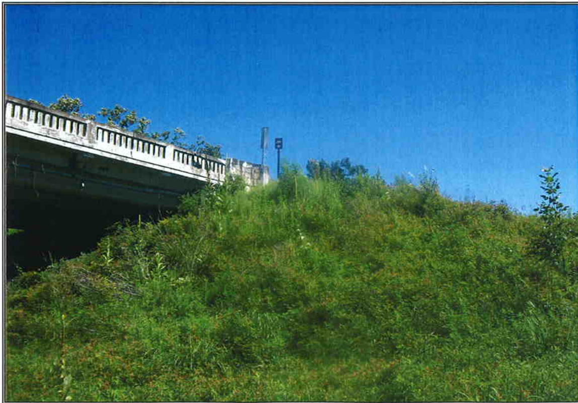
Looking at existing bridge end bent from proposed Bent 58 Centerline
