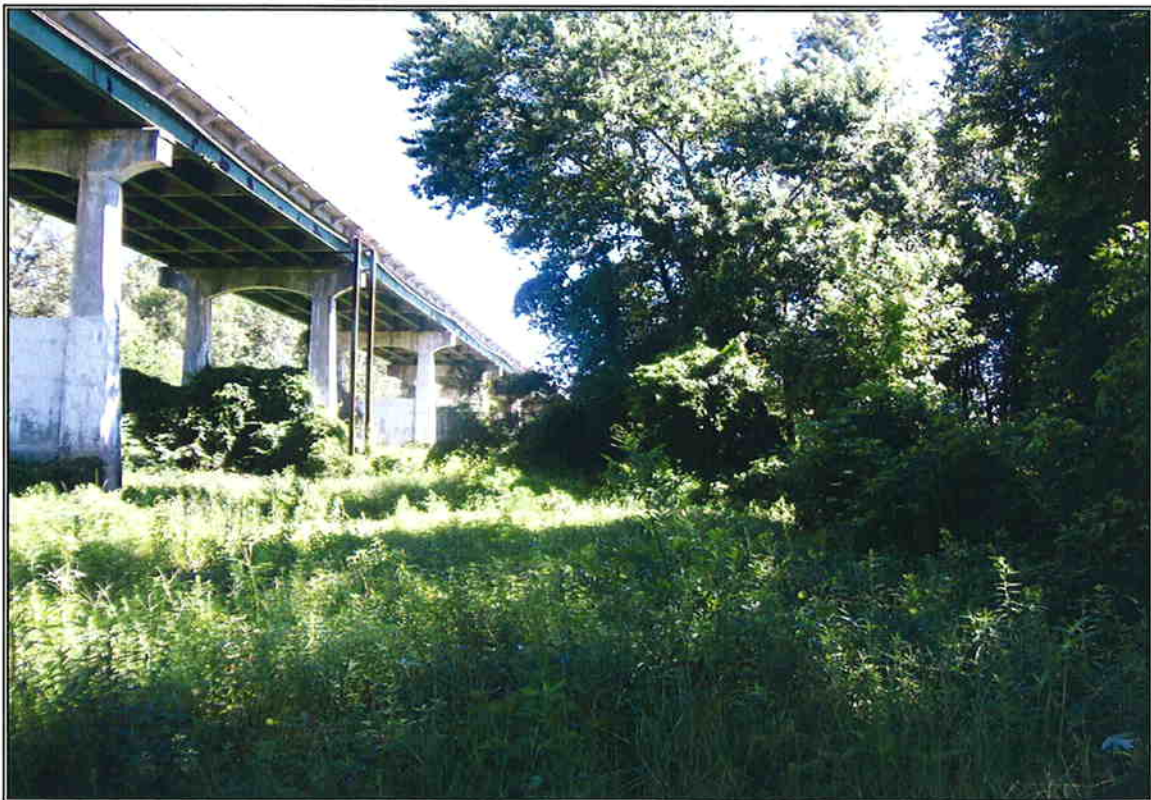
Looking in increasing station from proposed Bent 5 Centerline
