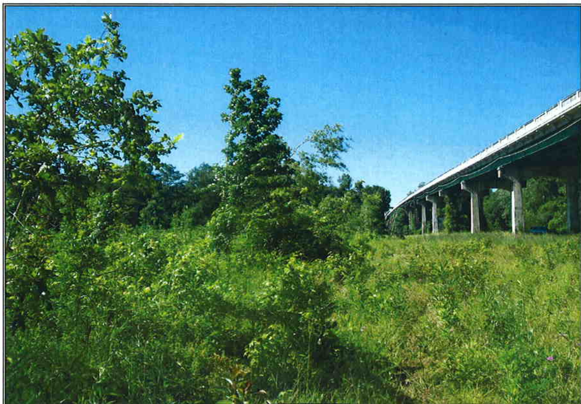
Looking in decreasing station from proposed Bent 13 Centerline
