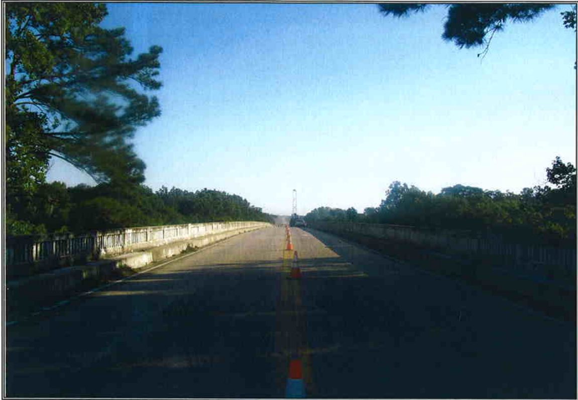
Looking in increasing station from existing bridge centerline at station 47+40
