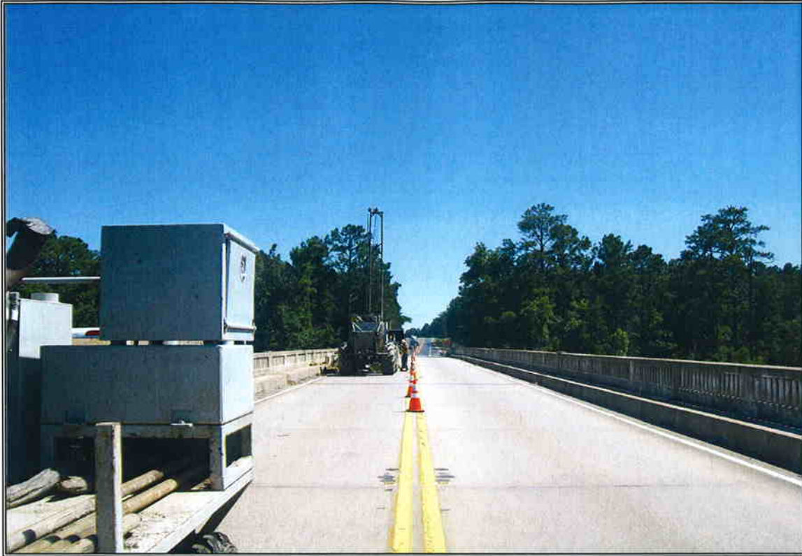
Looking in decreasing station from existing bridge centerline at station 51+60
