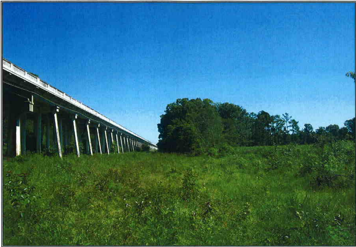
Looking in increasing station from proposed Bent 13 Centerline
