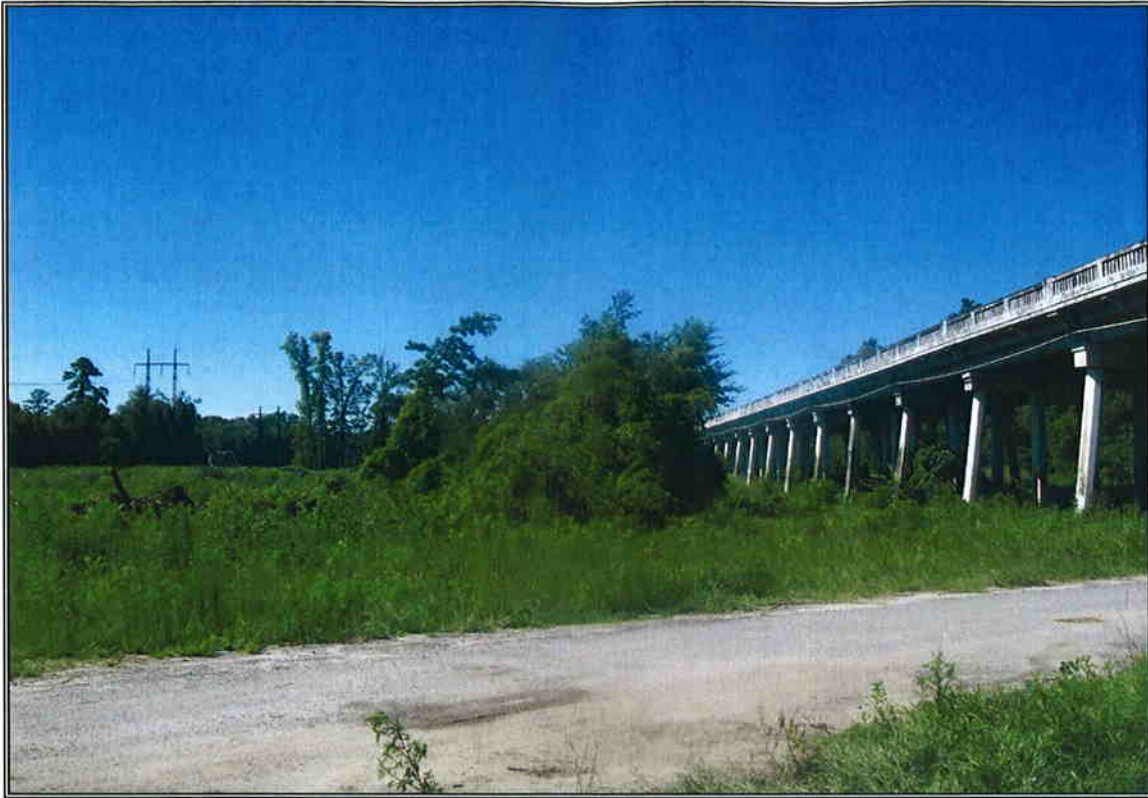
Looking in decreasing station from proposed Bent 58 Centerline
