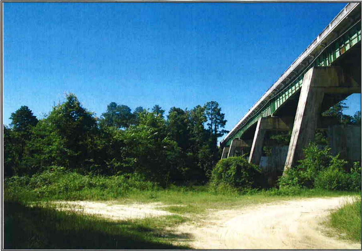
Looking in decreasing station from proposed Bent 5 Centerline
