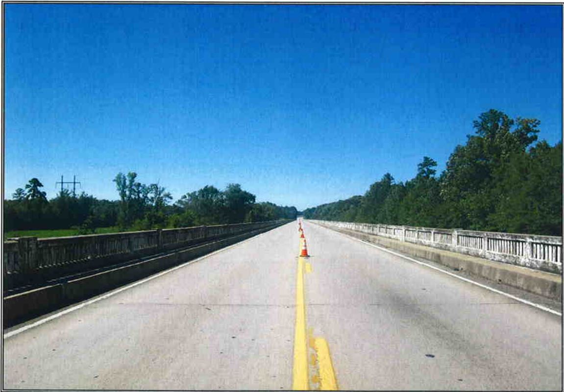
Looking in decreasing station from existing bridge centerline at station 88+20
