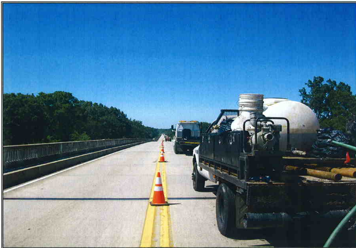
Looking in increasing station from existing bridge centerline at station 51+60
