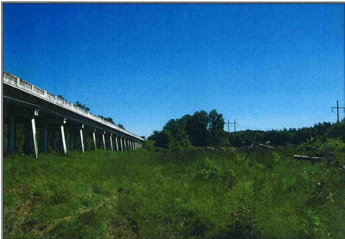
Looking in increasing station from proposed Bent 48 Centerline
