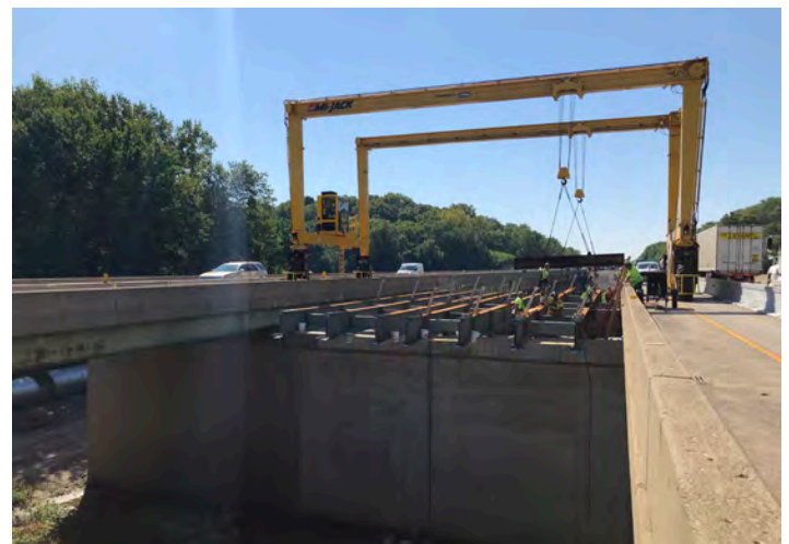
Mi-Jack Straddle Crane (Superior Project)
