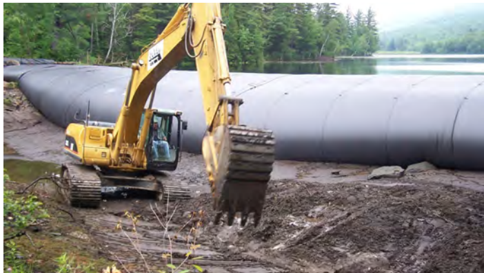
Example of Temporary Cofferdam
